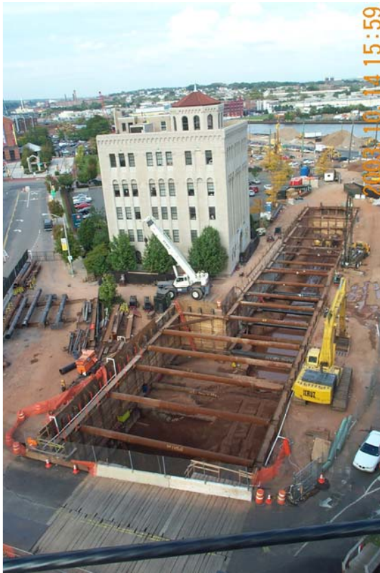
Photos taken in October 2003 show the excavation support and underpinning structures during the construction of the one mile extension of the Newark subway. At left: The temporary excavation support consists of a soldier pile and lagging wall and secant pile walls. Above: Because the tunnel passes under the PSE&G electrical vaults on Mulberry Street, these structures required underpinning protection during construction.
