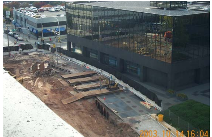
Photos taken in October 2003 show the excavation support and underpinning structures during the construction of the one mile extension of the Newark subway. At left: The temporary excavation support consists of a soldier pile and lagging wall and secant pile walls. Above: Because the tunnel passes under the PSE&G electrical vaults on Mulberry Street, these structures required underpinning protection during construction.
