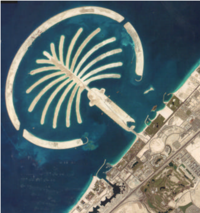
MRCE performed a geotechnical review of the design of the foundations for the Atlantis Development, a resort on created land offshore in Dubai. At left: Satellite image of the palm-shaped artificial island.
