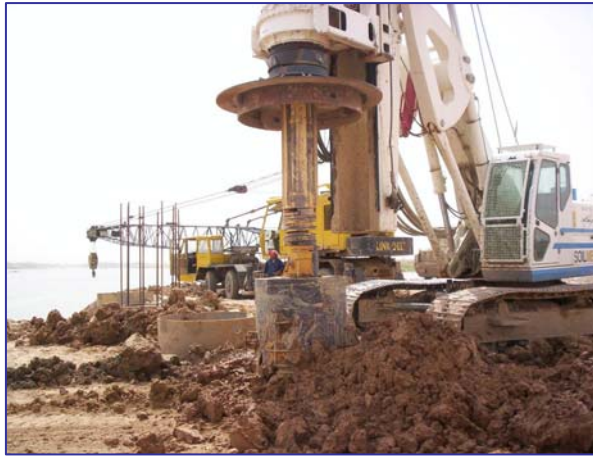
Left: Drilled piers during construction. Right: Aerial photo of the location for the Ramadi Bridge.
