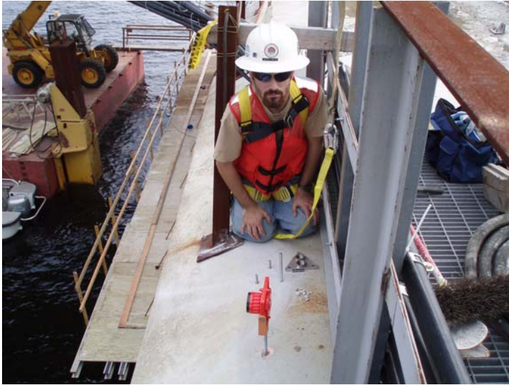
Above: Installing a tiltmeter on a bridge pier. Right: Drilling on the piers.
