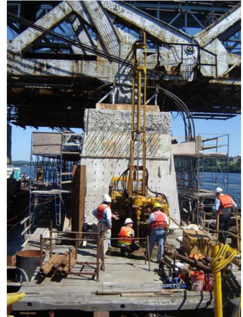
Above: Installing a tiltmeter on a bridge pier. Right: Drilling on the piers.
