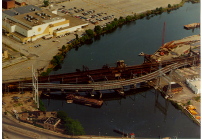
New run-around to bypass the Metro-North Peck Bridge at Bridgeport, CT.
