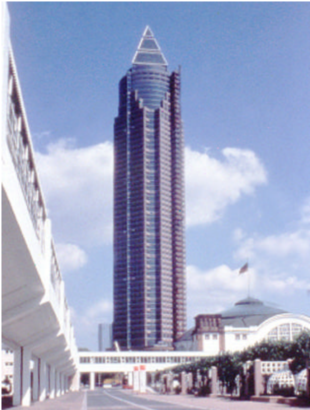
Completed MesseTurm building in Frankfurt.
