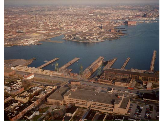
Above: Site prior to construction. At left: One high rise building under construction. Top center: the finished development with marina.
