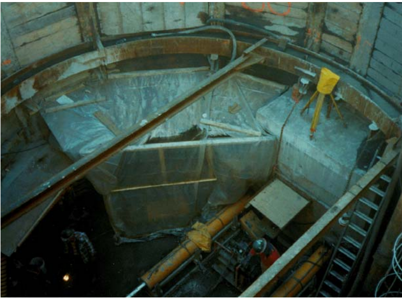
Above: The Jacking and Receiving Pit. At right: Intermediate Jacking Station.
