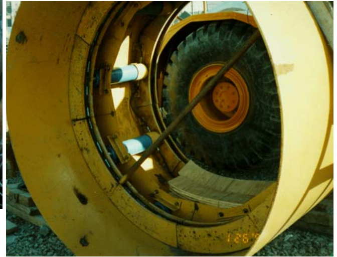
Above: The Jacking and Receiving Pit. At right: Intermediate Jacking Station.
