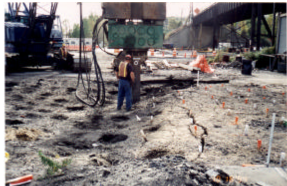
Both photos taken at Pier P2, with a view to the west. At left: Vibratory probe grid prior to the start of the densification. Note the close proximity to existing bridge. At right: Densification of the subgrade using vibratory probes.
