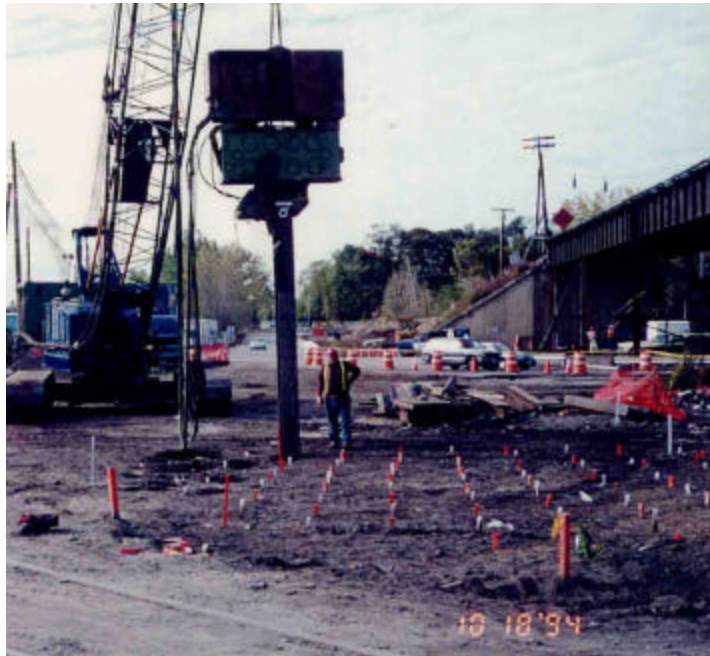
Both photos taken at Pier P2, with a view to the west. At left: Vibratory probe grid prior to the start of the densification. Note the close proximity to existing bridge. At right: Densification of the subgrade using vibratory probes.
