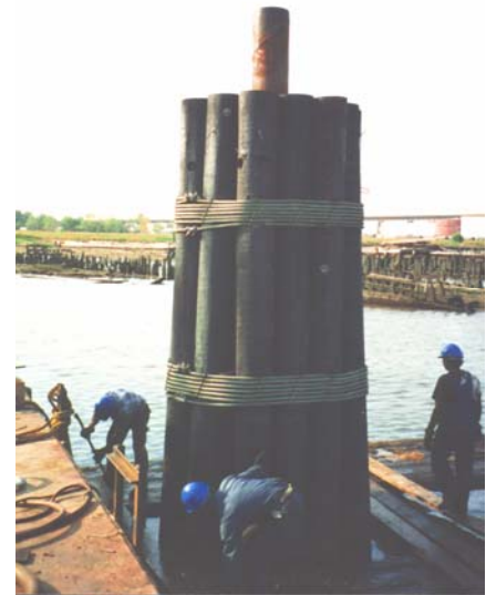
Upper Left: Steel walkway accesses the mooring clusters. Lower Left: MRCE-designed fender system facing the T-Head pier for The New Jersey Responder. Above: MRCE inspected the installation of the mooring clusters.
