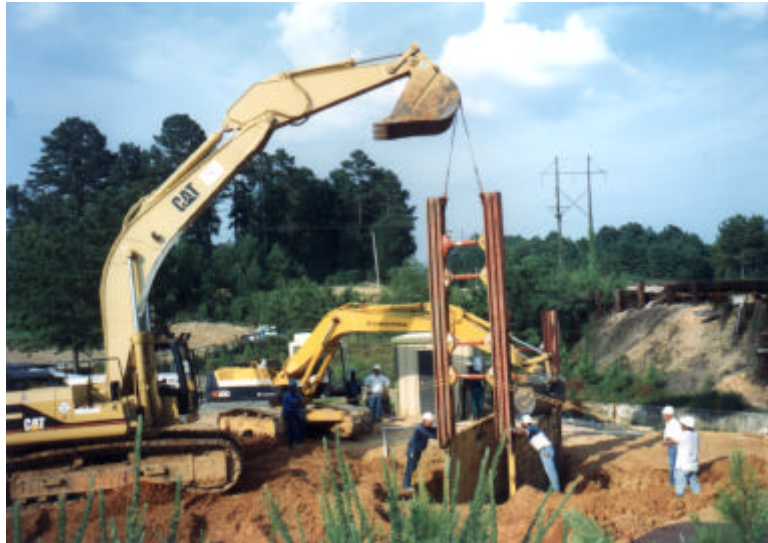
Construction of the replacement interceptor trench.
