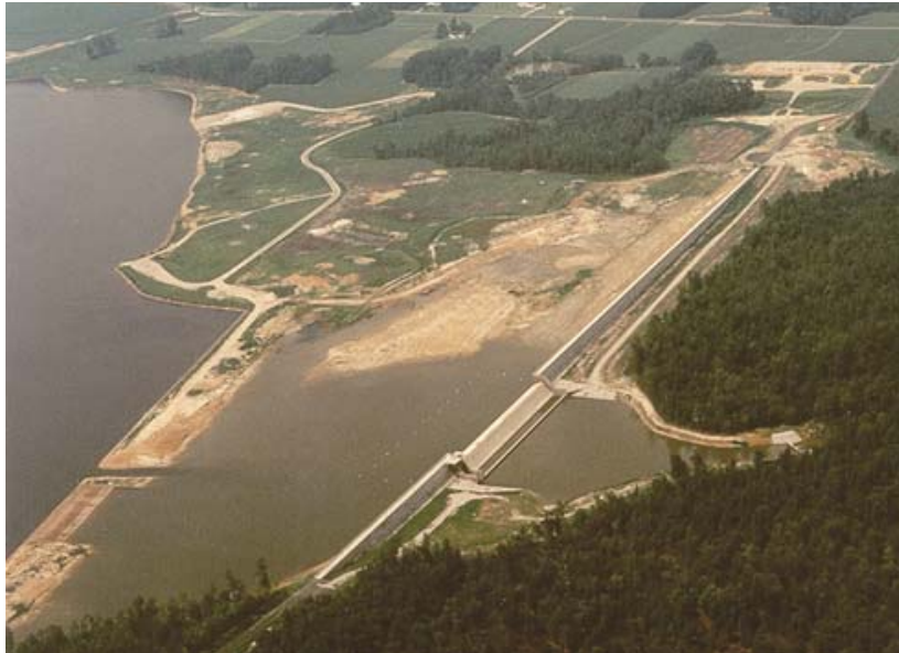
Aerial photo shows the previous 15-foot high dam on left, with the new 47-foot high dam at right.
