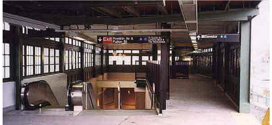
Above and at left: New entrance facilities and new entrance well.
