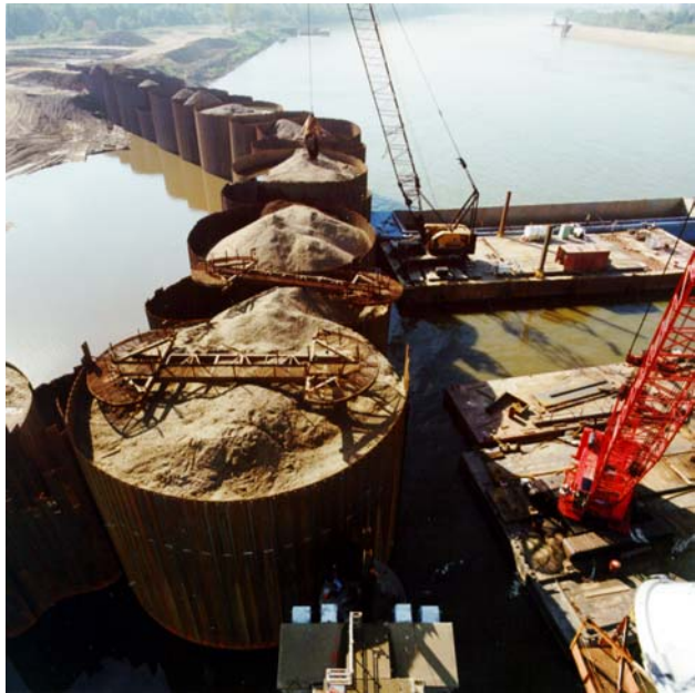
Photo of construction showing circular cells used (above and lower left), and view of Hydroelectric Plant where MRCE designed a cofferdam to protect the structure from possible flooding reaching a 65' head (lower right).
