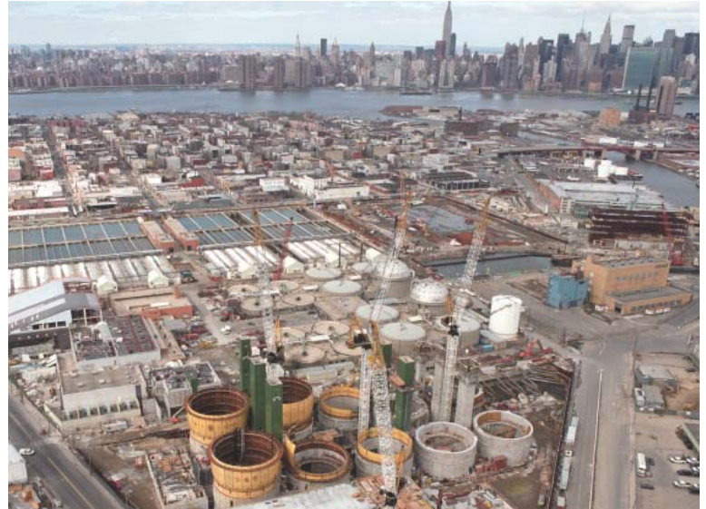
Above: Construction of the Digester Building includes 9 foot thick mat foundations, sheet walls with tiebacks and a raker-braced wall, all MRCE designs. At right: Looking southwest toward Manhattan, the digester tanks are under construction in the foreground of the photo taken in 2004. The eight digesters rest on 9 foot thick mat foundations.
