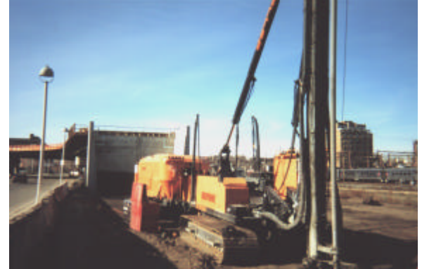
Above: The Light Rail System in operation at Exchange Place station. Right: Drilling and mixing equipment installing the soil cement columns in the Newport area of Jersey City, next to Hoboken and Long Slip channel. Behind the drilling equipment is the tanker where the injected cement is stored. The MRCE-designed abutment in the background supports a Wye shaped interchange with elevated steel bridge members.
