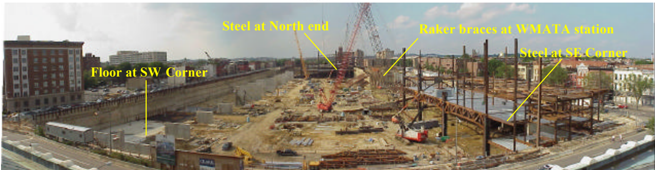
Upper left: Aerial view of completed convention center in 2003. Upper right: Cross-section of the convention center showing position of the subway and underground structures in relation to the building. Above: Convention Center site excavation taken from south end in July 2000.
