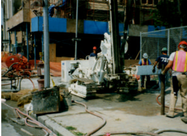
Deep soil grouting (above) during Phase I and placing the geogrid (at left) during Phase II of the reconstruction of St. Felix Street.
