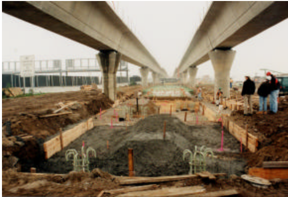
Above: Tunnel under the taxiway during construction. The excavation support system for the cut-and-cover tunnel under taxiways at JFK International airport is an MRCE design. Top Left: The construction on the Van Wyck Expressway progressing in June 2000. Lower Left: Superstructure construction at the airport.
