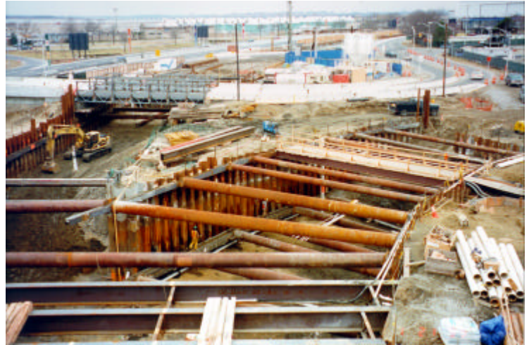
Above: Tunnel under the taxiway during construction. The excavation support system for the cut-and-cover tunnel under taxiways at JFK International airport is an MRCE design. Top Left: The construction on the Van Wyck Expressway progressing in June 2000. Lower Left: Superstructure construction at the airport.
