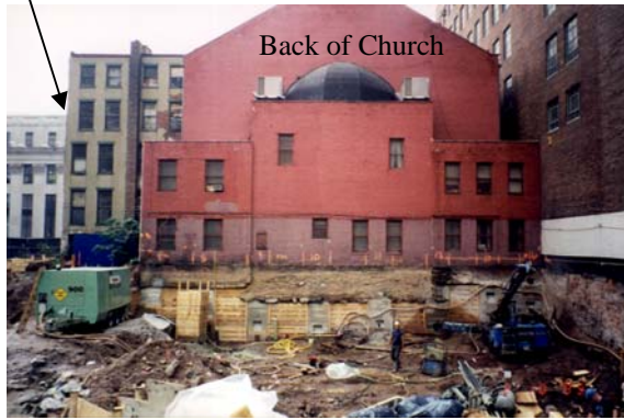
Top left: The completed theatre on 34 th Street. Lower left: Underpinning of the neighboring historic red church was required. Top right: Rock cut along 34 th Street. Lower right: Close-up of underpinning showing support buttons.
