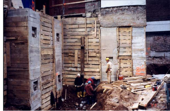
Top left: The completed theatre on 34 th Street. Lower left: Underpinning of the neighboring historic red church was required. Top right: Rock cut along 34 th Street. Lower right: Close-up of underpinning showing support buttons.
