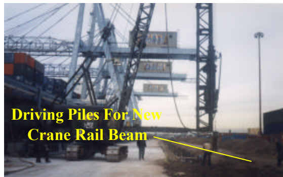
Lower Left: Driving piles for the new crane rail beam. The remainder of the photos on this page and the next show some completed projects in January 2004.
