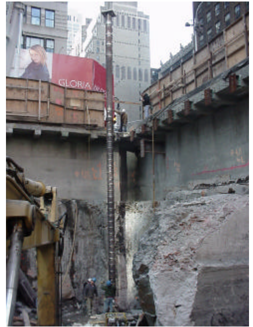
Upper left: Location map showing the 4 buildings for which MRCE performed geotechnical investigation. Center top: Artist rendering of completed Times Square Tower building. Above: lifting and setting the caisson core. Center bottom: installing column sections. Lower left: MRCE inspector on site.
