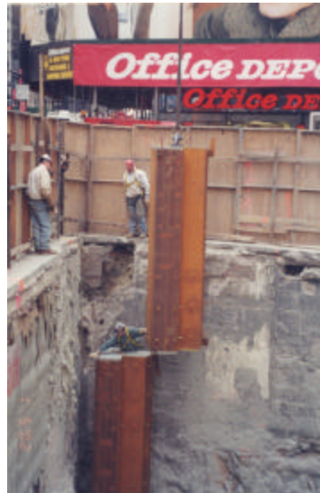
Upper left: Location map showing the 4 buildings for which MRCE performed geotechnical investigation. Center top: Artist rendering of completed Times Square Tower building. Above: lifting and setting the caisson core. Center bottom: installing column sections. Lower left: MRCE inspector on site.
