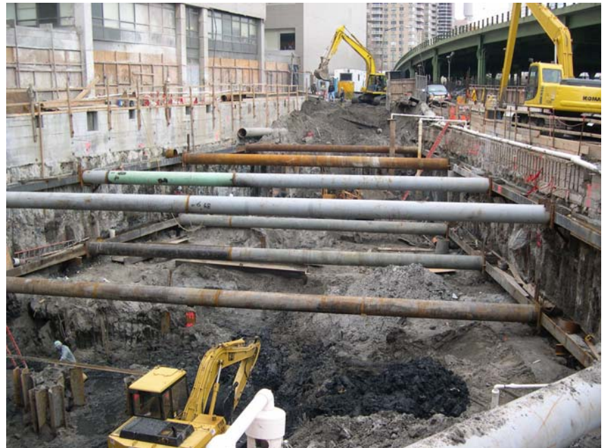
Above: Completed building with soils showing complicated underground. MRCE has performed over 50 projects for NYU Medical Center over the years. The new Smilow Research building is one of the most recent. At right: Excavation of basement for this constrained site. Note adjacent buildings on left and FDR Drive on right.
