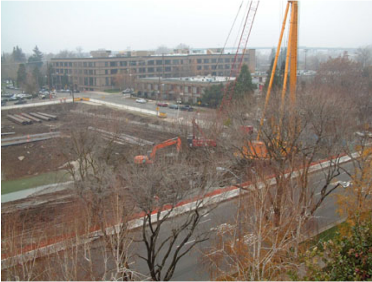
Above left: Artist's rendering of the completed building. Lower left: Largest triple auger rig used in the USA was imported from Japan by contractor for this project. Mast height is 118 feet. Above: Placing steel sheet pile into the upper portion of the soil-cement-bentonite mix. Sheet piling was braced with tiebacks for excavation support.
