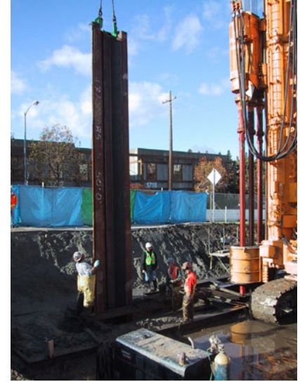
Above left: Artist's rendering of the completed building. Lower left: Largest triple auger rig used in the USA was imported from Japan by contractor for this project. Mast height is 118 feet. Above: Placing steel sheet pile into the upper portion of the soil-cement-bentonite mix. Sheet piling was braced with tiebacks for excavation support.
