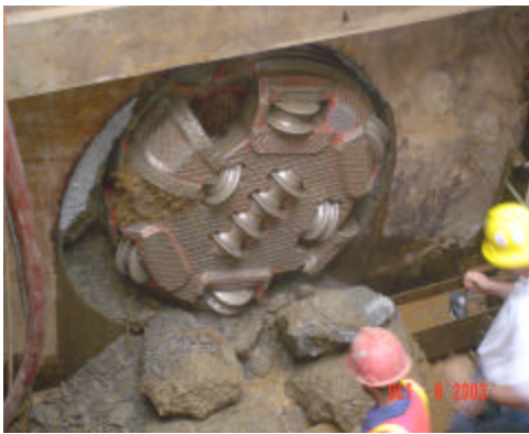
Above left: Tight site; maintaining one lane of traffic during construction. Lower left: TBM holing through at Shaft 6. Above right: Between shoves at Shaft 5.
