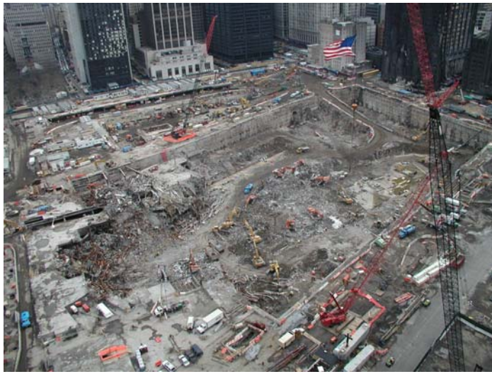
Above: Site overview taken 2/4/02 during tieback reinstallation. At right: MRCE engineers conduct load tests on tiebacks. At left: MRCE engineers performed a condition survey of the damage on the 1/9 and N/R subway lines under and near the WTC site following the collapse of the towers.
