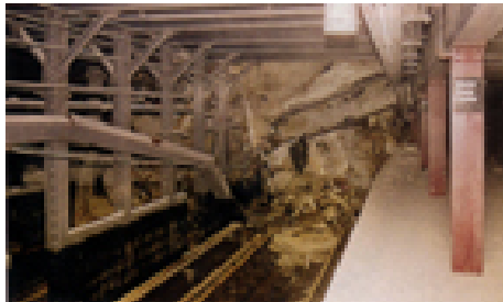
Above: Site overview taken 2/4/02 during tieback reinstallation. At right: MRCE engineers conduct load tests on tiebacks. At left: MRCE engineers performed a condition survey of the damage on the 1/9 and N/R subway lines under and near the WTC site following the collapse of the towers.
