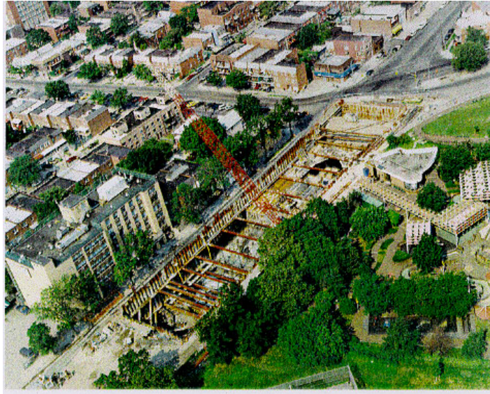
Construction of the Flushing Bay Corona Avenue Vortex.
