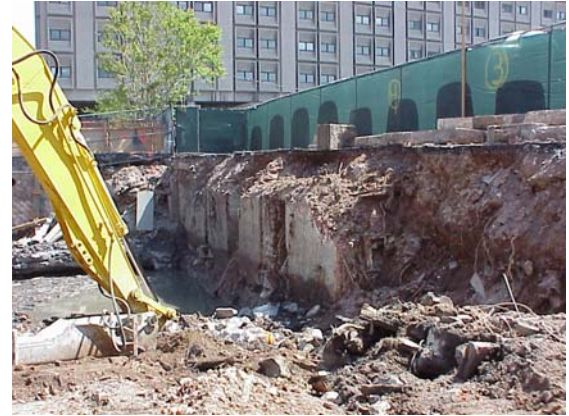
Left: Installing sheet piling excavation support. Above: Excavating previous structures.
