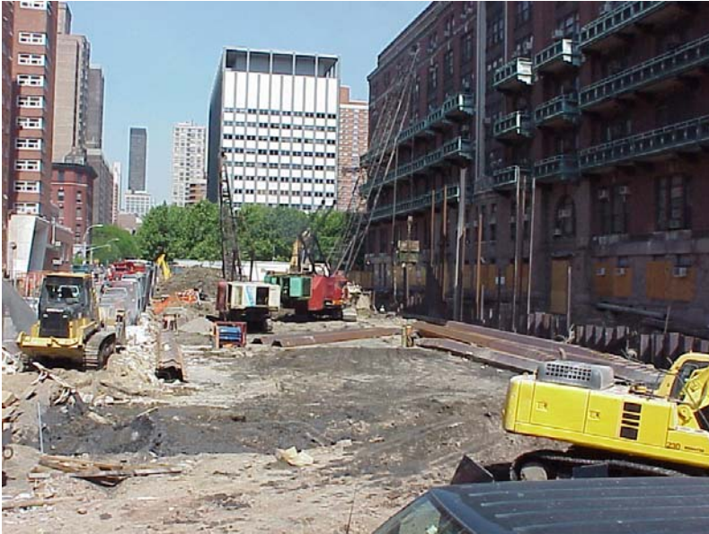
Left: Installing sheet piling excavation support. Above: Excavating previous structures.
