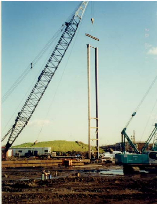
Above: Lowering typical upper frame assembly for slurry wall panel. Upper right: Site activity in December, 2002. Lower right: Slurry panel excavation with mechanical clamshell bucket.
