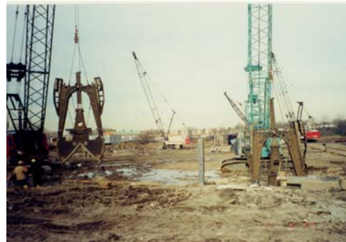
Above: Lowering typical upper frame assembly for slurry wall panel. Upper right: Site activity in December, 2002. Lower right: Slurry panel excavation with mechanical clamshell bucket.
