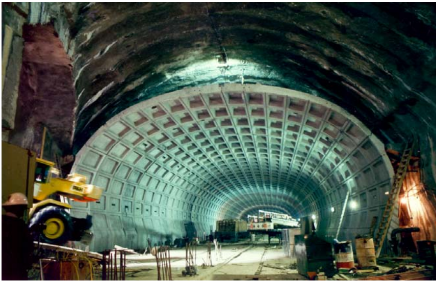
At left: Installation of a tunnel liner in WMATA station at Dupont Circle. Right: Completed Glenmont Station.
